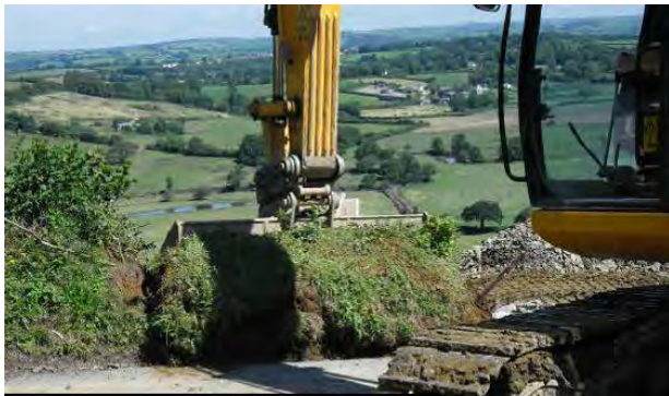
Removing slab of hedgerow ground flora
